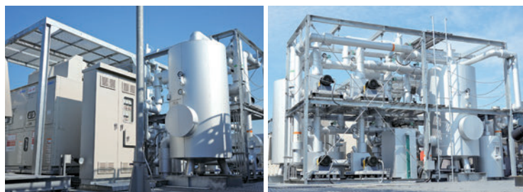
Heat recovery heat pump system
