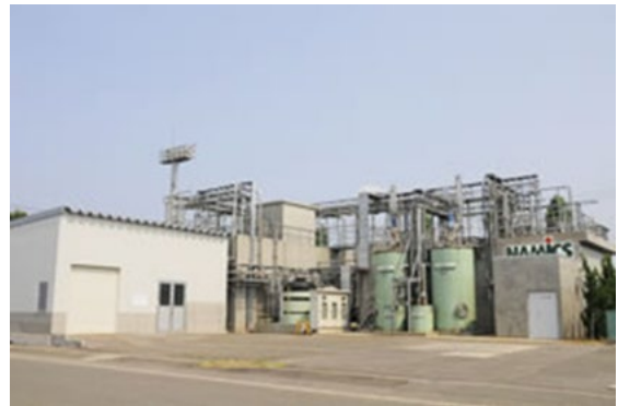
Wastewater treatment facilities (Head Office/Factory)
